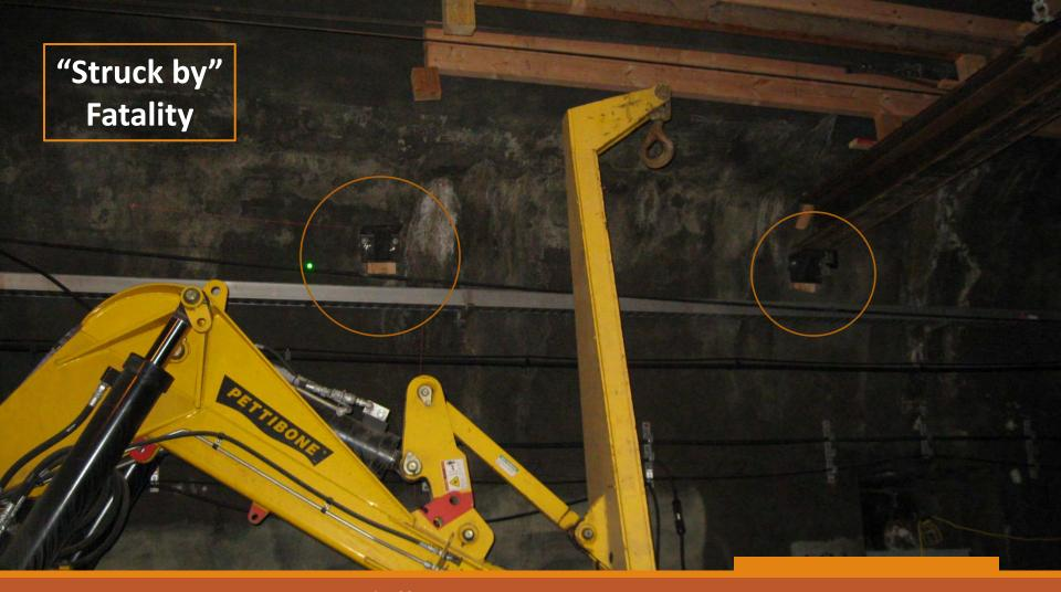
An employee was fatally injured when he was struck by an approximate 22.5-foot long, 1.2-Ton Steel Beam while walking out of the tunnel at the same time a slow moving Rail Crane was traveling into the tunnel pushing two loaded flat railcars with the extendable hydraulic boom attachment in the upward position. A collision between the boom and the beam knocked the beam off of its steel support brackets causing the beam to fall and strike the employee upon the head area.
